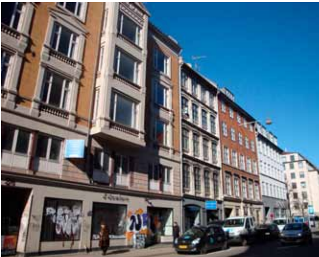
Facader mod Store Kongensgade.
