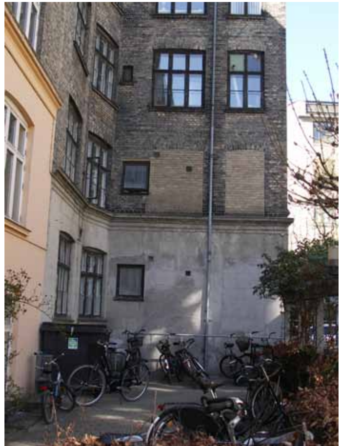
Facade mod gård
