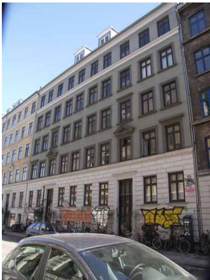
Facade mod gade
