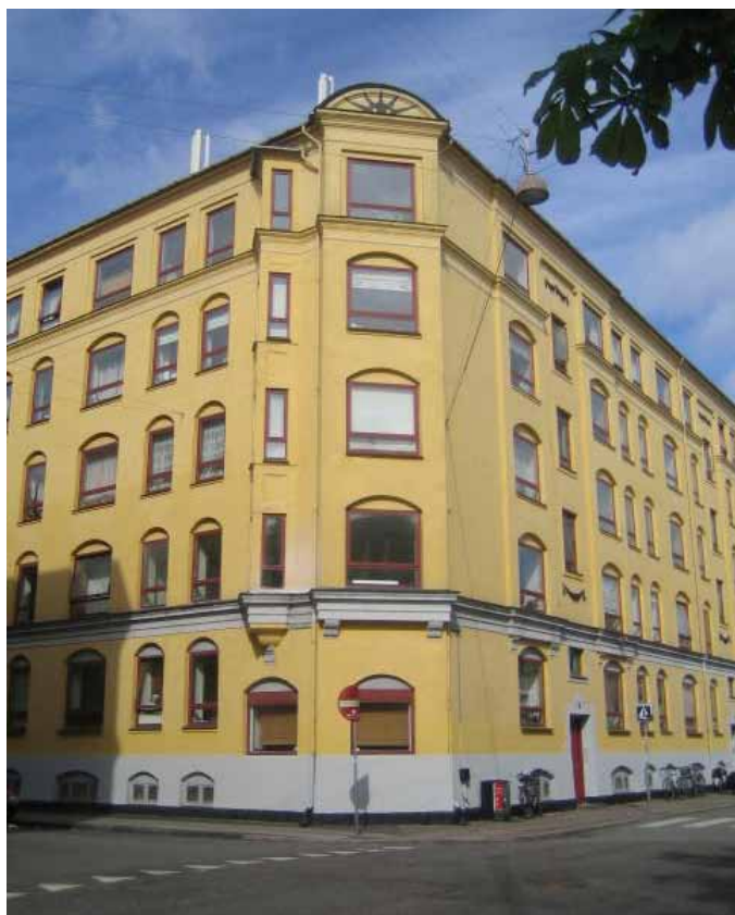
Facade mod gade
