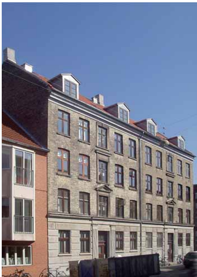
Facade, Sverrigsgade 6A-6B
