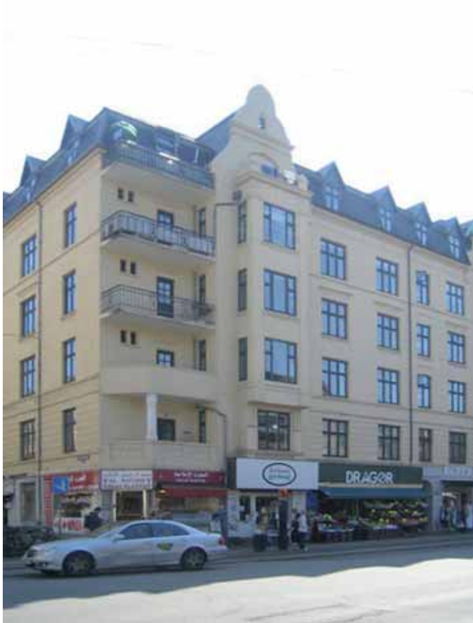
Facade mod Amagerbrogade
