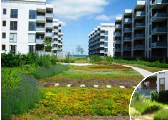
Underground garage, Holbæk
