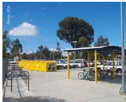
Bicycle parking and storage facilities
