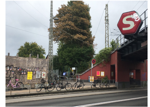
ill.16c Vanløse station is a source of potential visitors and the raised tracks offer a clear view of the site when you pass by with the train.
