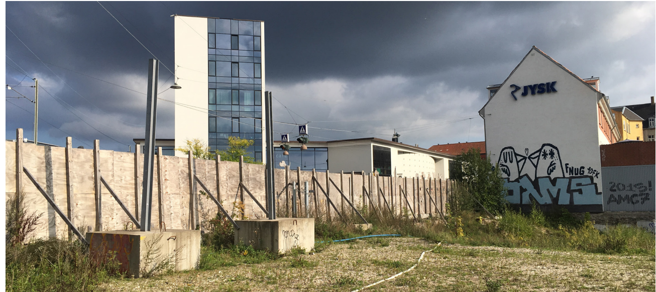
ill.27b The fence from the site
