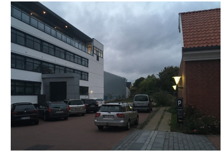
ill.17d Julie Arenholts Vænge street view towards the site from the south
