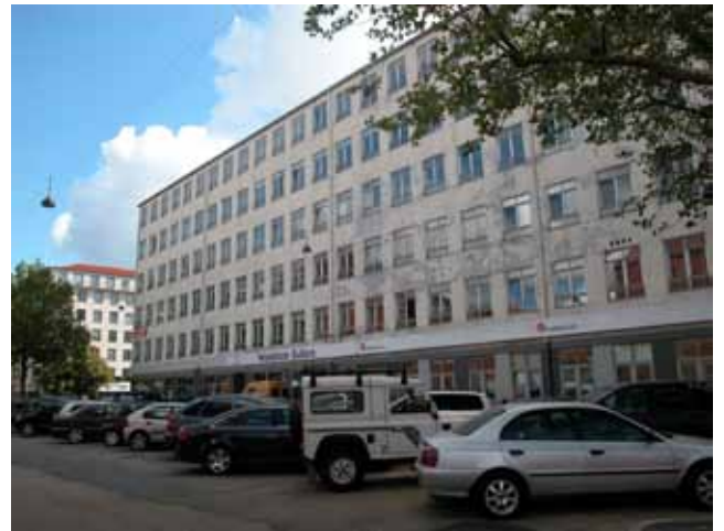
Facade mod Borgergade ("Borgergadehus").
