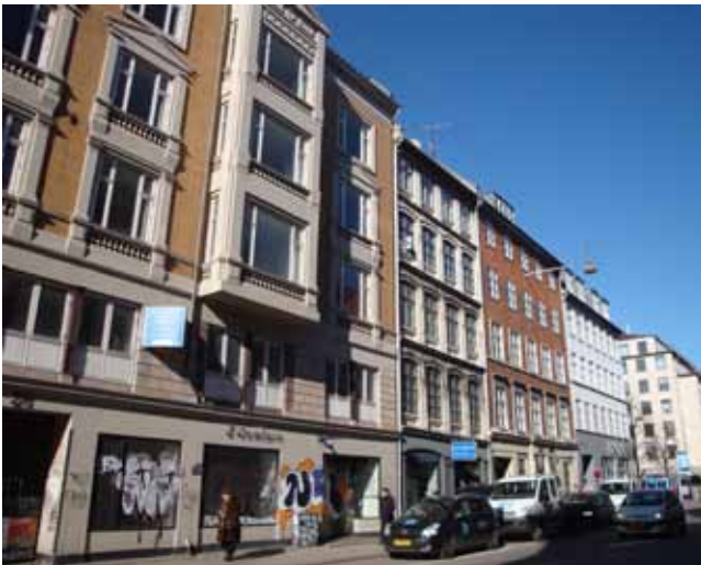
Facader mod Store Kongensgade
