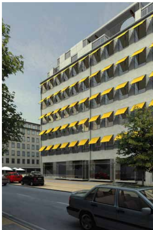
Ny facade "Borgergadehus".
