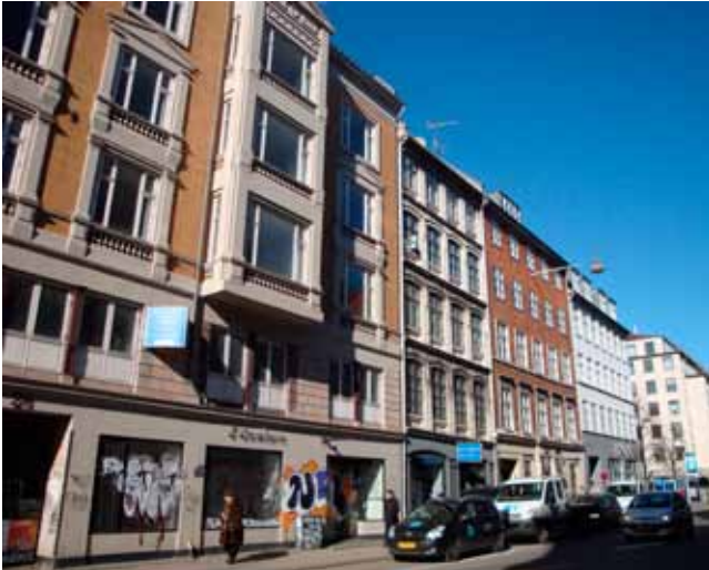
Facader mod Store Kongensgade.
