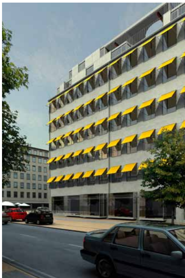
Ny facade "Borgergadehus".
