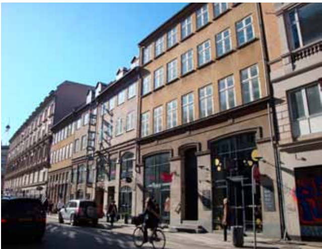
Facader mod Store Kongensgade.
