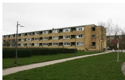
Facade mod have
