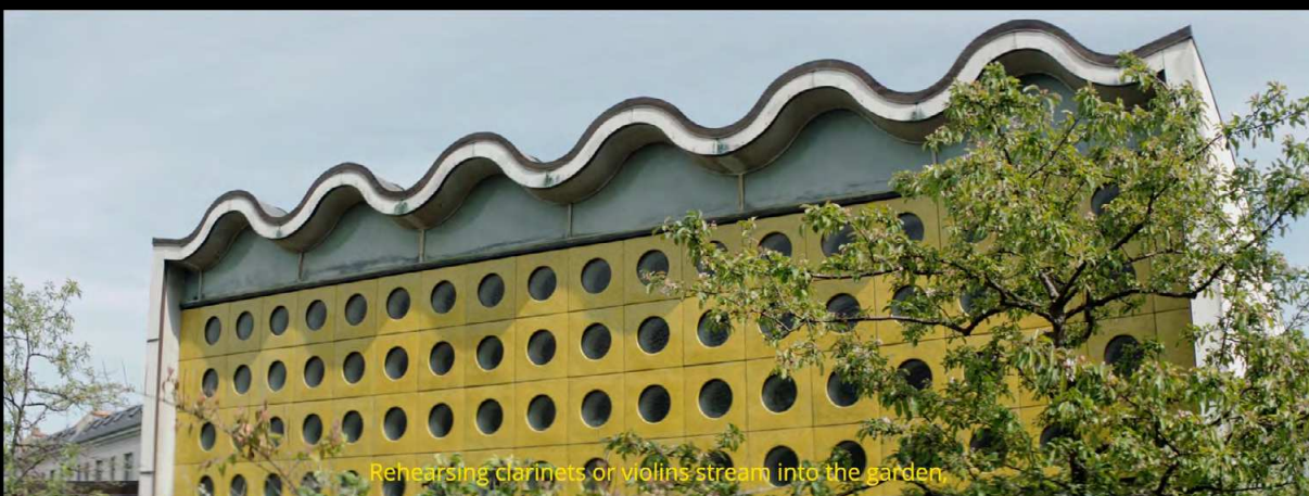
they're connected to rooms below the organic roof
