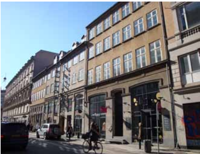
Facader mod Store Kongensgade
