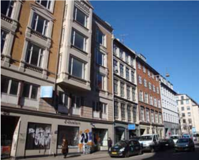
Facader mod Store Kongensgade
