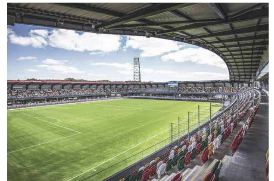
Silkeborg Stadion, Sweco Architects
