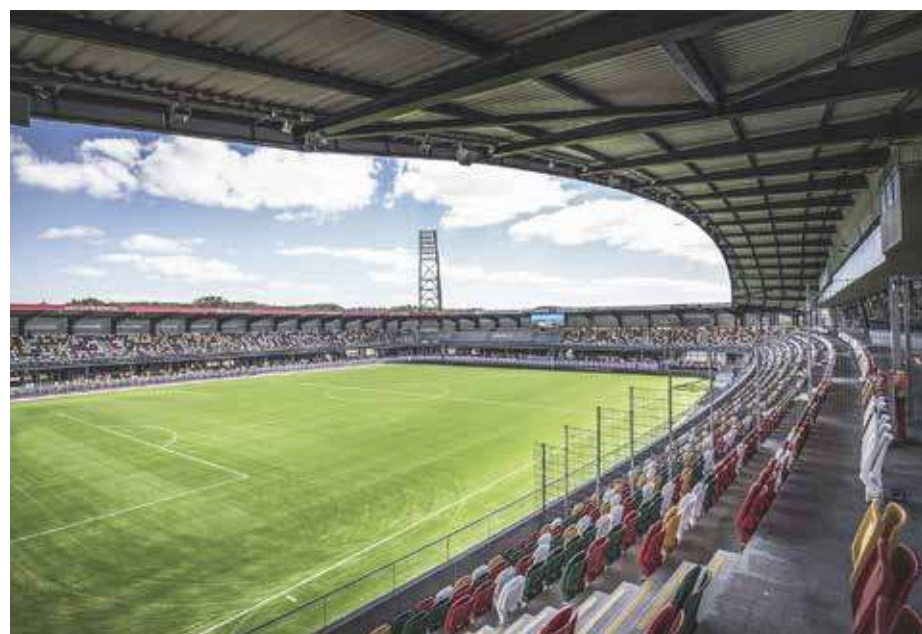
Silkeborg Stadion, Sweco Architects
