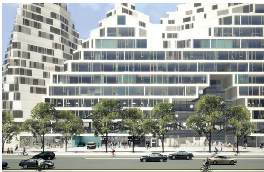
Batteriets facade mod Njalsgade (illustr. BIG)
