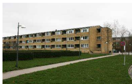
Facade mod have
