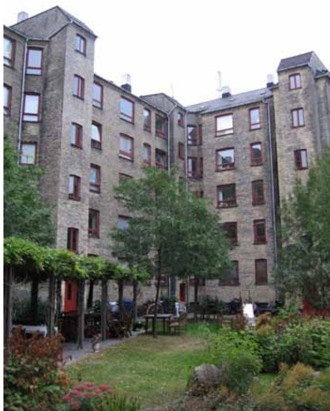
Facade mod gård
